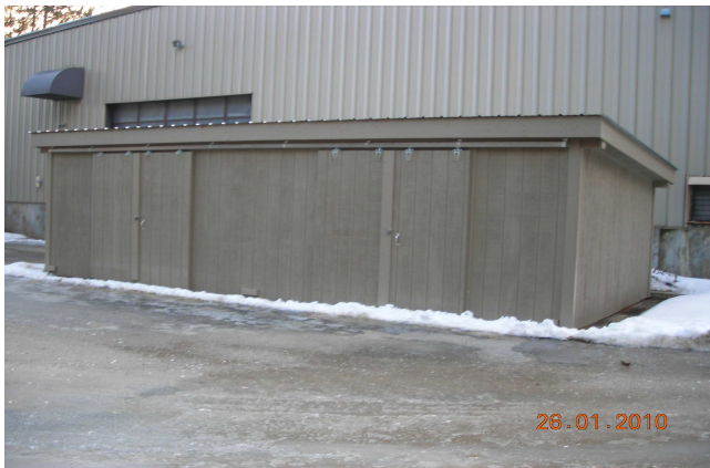
Sign storage shed built with help from Merrimack County Inmates.
