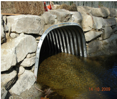
Mason Hill Road culvert
