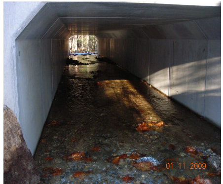
Box culvert installed on Horne St.
