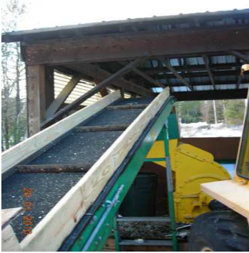
Rebuilt conveyer at the Transfer Station donated by Warner Power.
