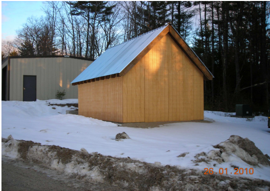
Parks & Recreation storage shed built with help from Merrimack County Inmates.
