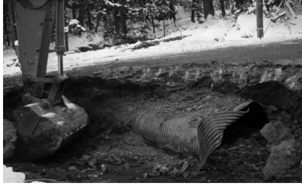
Culvert During Repair
